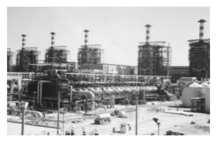
**FIGURE 20.6.2** One of the six units of the 346,000 m<sup>3</sup>/day MSF desalination plant Al Taweelah B in Abu Dhabi, United Arab Emirates. (Courtesy of Italimpianti S. p. A.) It is a dual-purpose plant, composed of six identical power and desalination units. Five of the six boilers are seen in the background. The desalination units were in 1996 the largest in the world. They have 17 recovery and 3 reject stages and a performance ratio (PR) of 8.1. The plant also produces 732 MWe of power.
