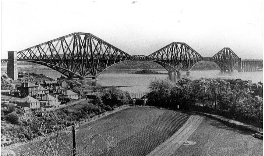
8.2 The Forth railway bridge.
